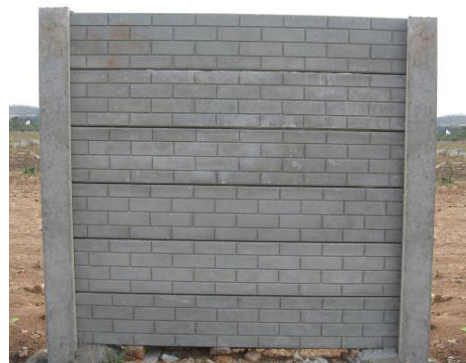
RectaBrick Plus Precast Compound Wall moulds
